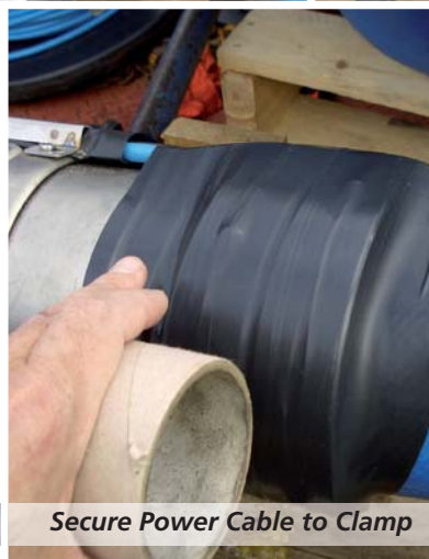
3. Secure Coupling
